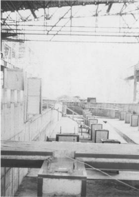
STEEL WORKS PLANT REINFORCED CONCRETE FOUNDATIONS, NOVOKUZNETSK - RUSSIAN F.
